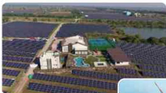
Sudi Iconic Solar Park, Bharuch
