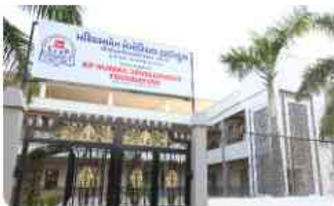
KP Human renovated Mariyamben Memorial High School
